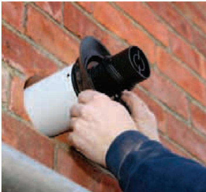
Installation of a Greenstar Oilfit RS flue system
