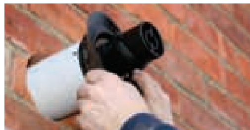
Installation of a Greenstar Oilfit RS flue system
